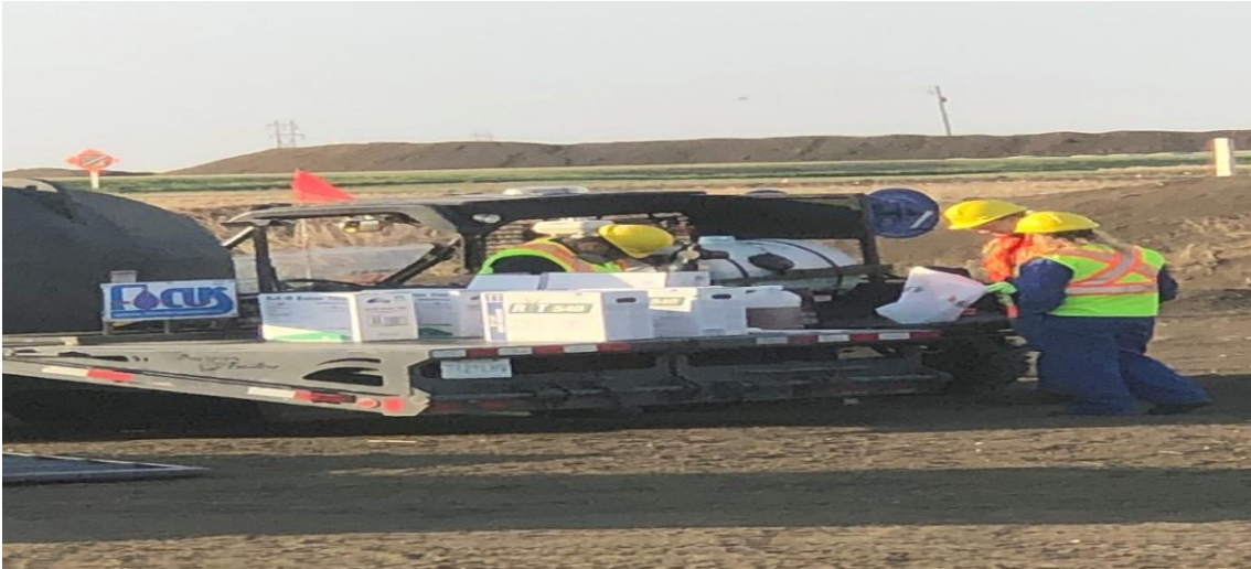
Mixing chemicals to spray @ KP 527+900.
