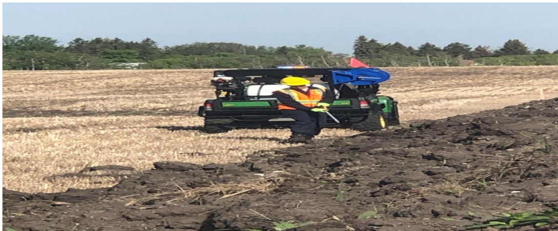
Hand spraying along top soil pile @ KP 784+000.
