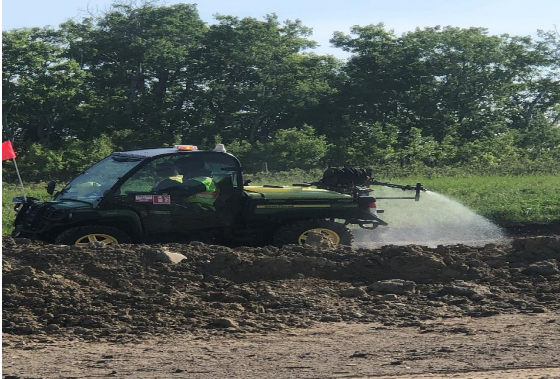
Crew spraying from mobile unit. KP 784+000.
